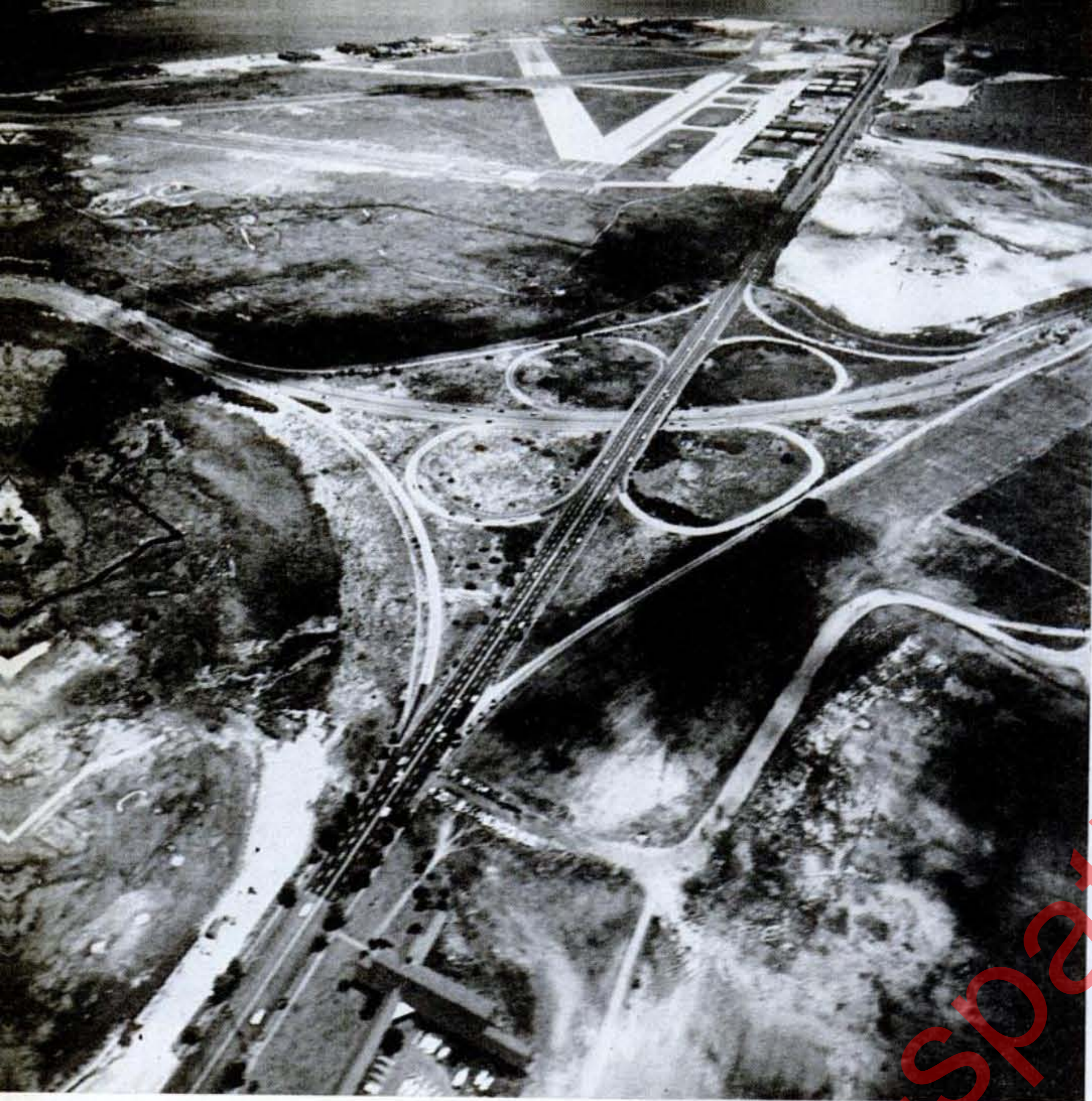
DESTINATION. Floyd Bennett Field ( top ), is photographed by portside camera as the jet circles for its final approach. Cloverleaf connects Brooklyn's Flatbush Avenue ( foreground ) with Belt Parkway.
